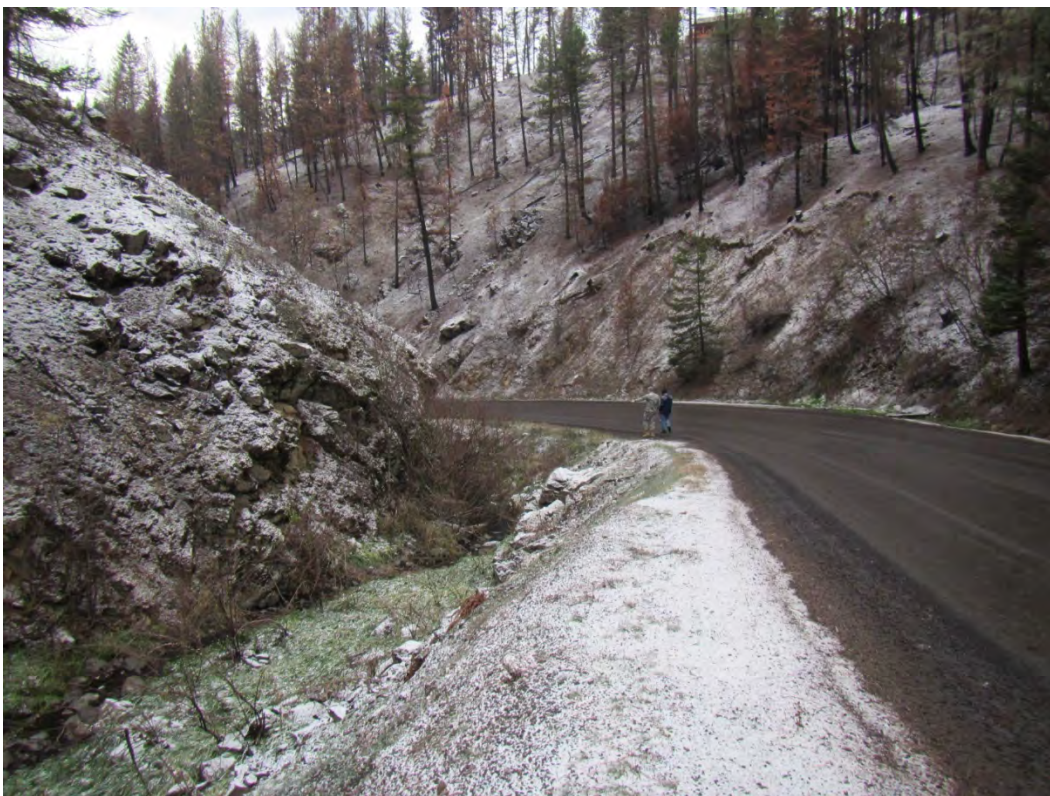
Photo 6. Upstream of the Adams Grade/Glenwood Road intersection. Potential flooding of the road is possible at this location where the channel could easily plug.
