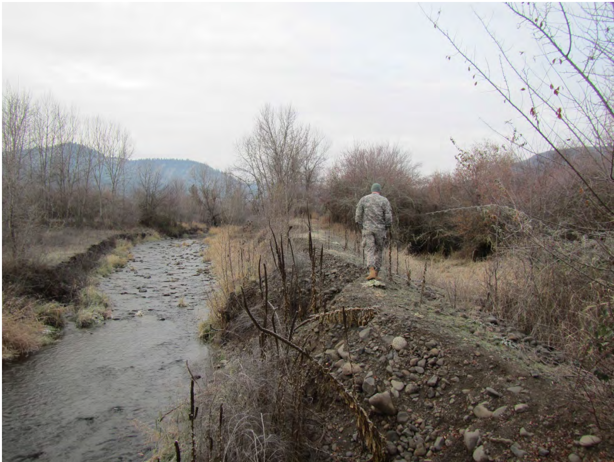
Photo 5. Eroded left bank levee upstream of the railroad bridge in Kamiah.
