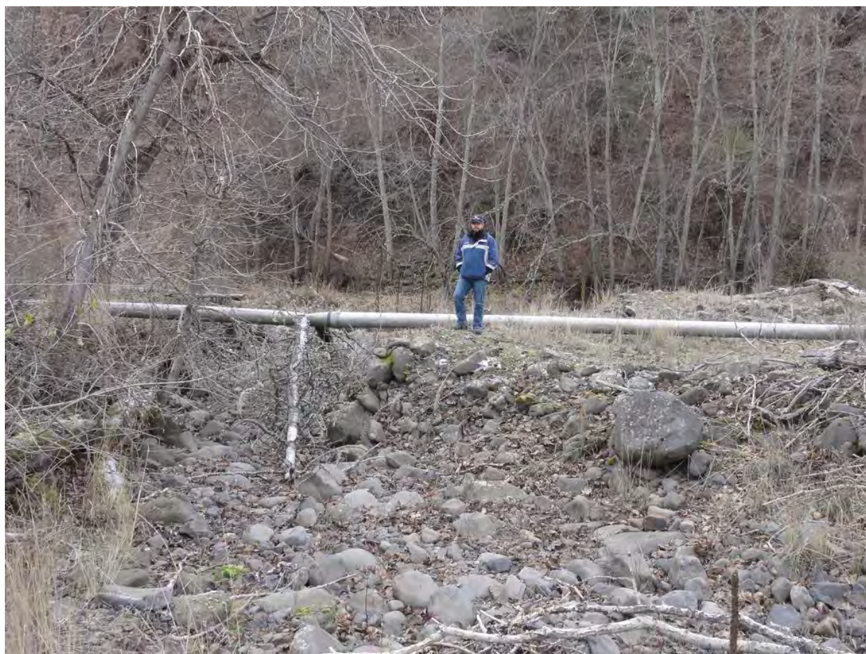
Photo 1. Restricted Suzie Creek channel near confluence. The water pipe and downed tree have the potential to catch debris and exacerbate the constriction at the mouth of Suzie Creek.
